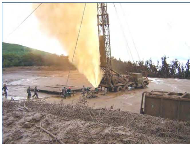
Figure 3-1 Inland well blowout while being decommissioned. Source: www.archive.epa.gov
